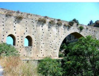
The aqueduct spans the valley and the stream in two superimposed arcs, here seen from the road towards Spília (Picture left). The picture right shows the "backside" from the way through the aqueduct. The lower wall strength is approximately 4 meter, the upper approx. 2 meter, where the upper part of both sides (with appropriate caution) is accessible. The countless niches serve as refuge and breeding cave for the neighbouring Jackdaw colony and pigeons.
