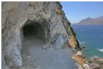
The flashlight is needed for exploring the approximately 2 meters wide, but only about 1.60 metre high tunnel. I have lighted the rock walls and did not discover a single blast; this passage was therefore worked by hand out of the mountain.
