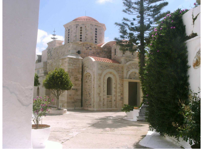
The reconditioned church in the monastery inner court
